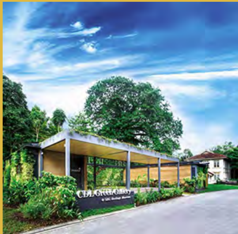
The CDL Green Gallery showcases two innovative green features incorporated for the first time in Singapore – Hempcrete, an eco-friendly biomaterial, and a prefabricated modular construction system which is easy-to-build and has a lower environmental impact.
