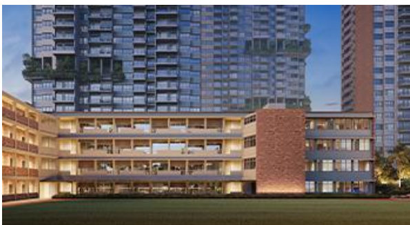
Part of the former Upper Thomson Secondary School has been conserved and converted into 32 homes and the Springleaf Club.
