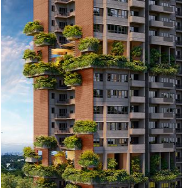
The 10 Sky Terraces can be found across the five residential towers, providing green spaces for residents.
