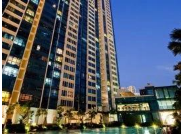
City Square Residences is a freehold condominium development with 910 units. The development has received accolades including the BCA Construction Excellence Awards, BCA Construction Productivity Award (Gold), and BCA Design & Engineering Safety Excellence Awards.
