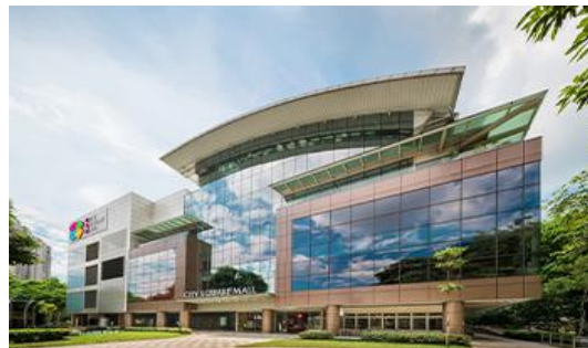
City Square Mall today reflects the district's transformation while continuing its long tradition as a gathering place for the community.
